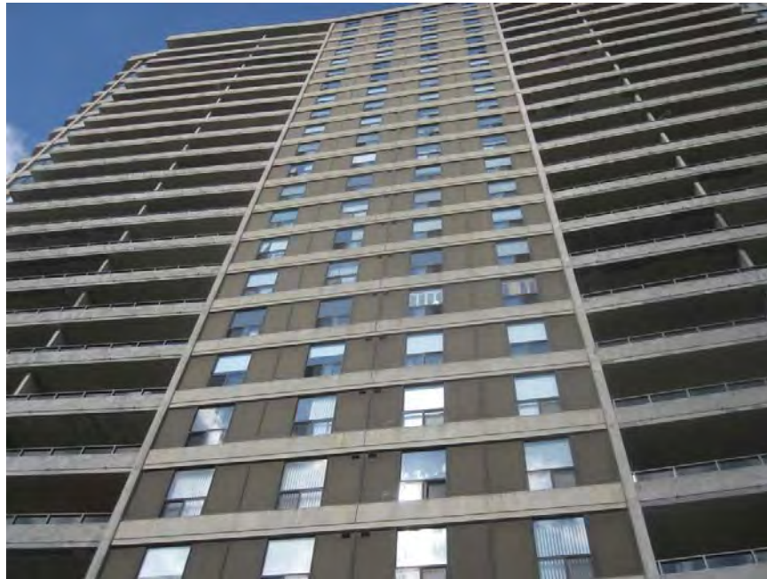
Photo 1: Punched windows and exposed metal wall panels on the West elevation.
