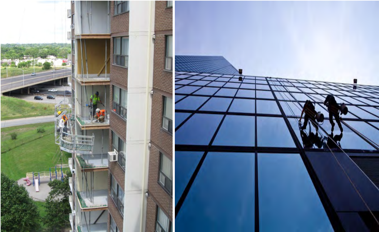
Photo 1.: Suspended Access Equipment – Swing Stage (left) and Bosun's Chair (right)
