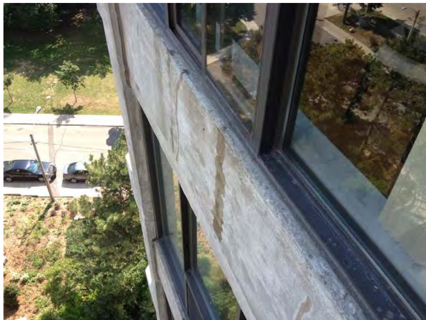
Photo 4: Concrete cladding panels are located below punched windows.
